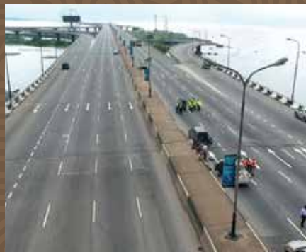
Third Mainland Bridge
